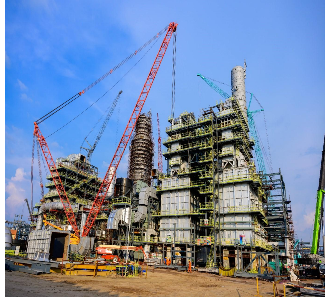
HRRL Project, Rajasthan
