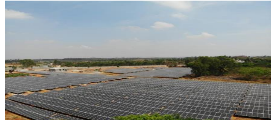
Solar Panels at HRGRDC, Bengaluru
